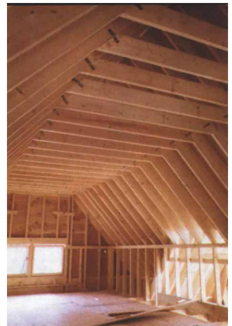
The shape revealed. The project began with standard gable roof framing. Flush cross ties (photo above) secured with metal plates roughed out the shape of the barrel vault. Plywood gussets (photo below) provided the final shape. They were screwed to the rafters.
