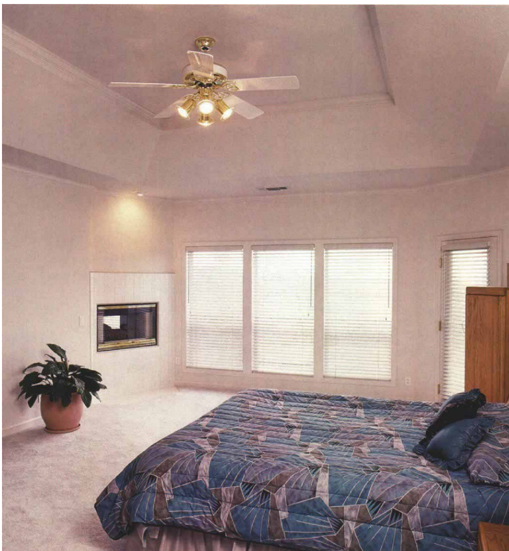
One big coffer. Soffits girdle this bedroom to support angled coffer framing. A single, recessed ceiling coffer is the result. Photo by Scot Zimmerman.
